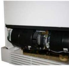
10 Connect power and remote humidostat wires.
